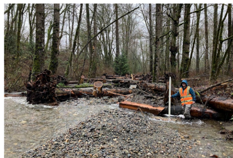
As-built condition and post flood event sediment accumulation at Swan Creek. Photo courtesy of Natural Systems Design
