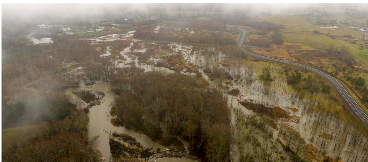
Lower Dungeness River Floodplain Restoration Project during the December 2025 floods. Photo Courtesy of Clallam County
